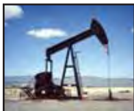
Down Hole Instrumentation
