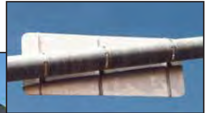
Mast Arm Sign Installation
