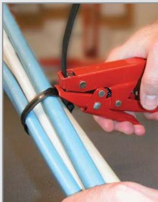
Tighten the tie till complete fixing of the cables.
